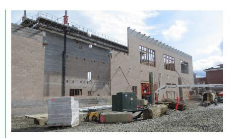
Work is progressing on the New Gym and we are beginning to close in the exterior. This will allow temporary heat and interior finishes to begin in all areas throughout the building. Roofing at the New Gym area will continue as weather permits. The New Theater CMU walls are complete and structural steel erection has begun and will continue throughout the month.
